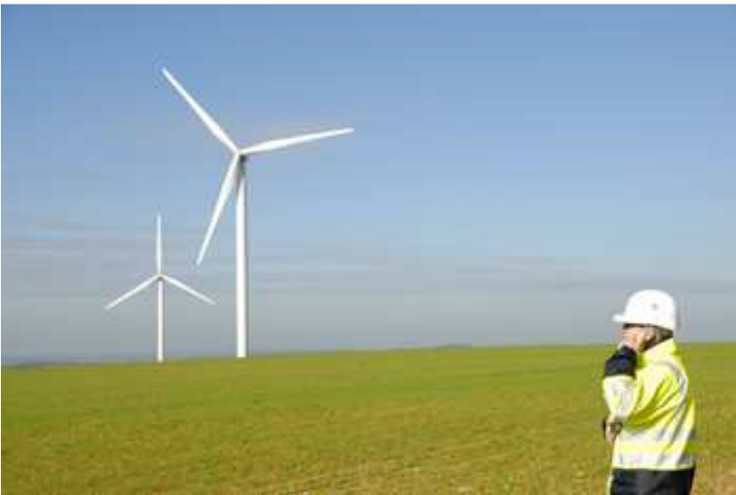
43. Energy Operations, Optimisation and Maintenance
