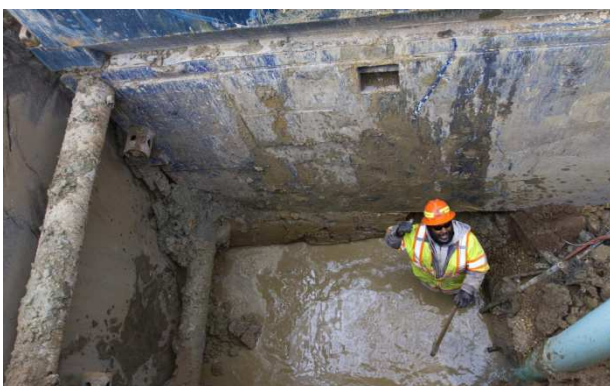
41. Sanitation and Air Pollution during Construction
